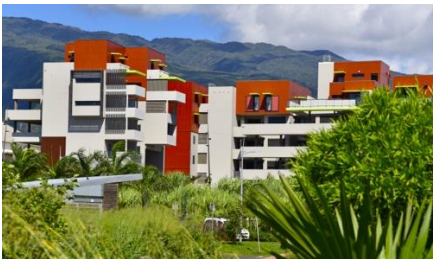
Anthurium (63 housing units and 107 parking spaces)
